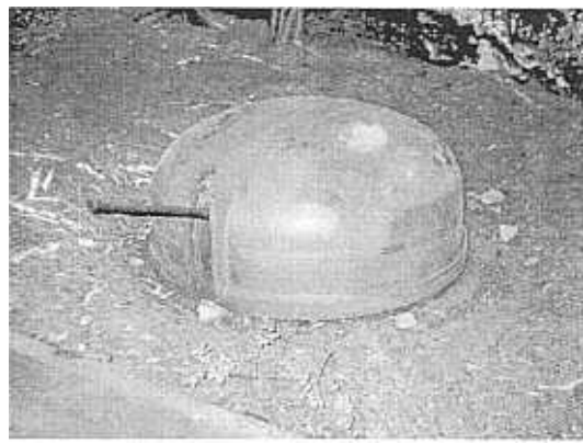
Bunker with steel cupola armed with a heavy Browning M2 machinegun - the oldest part of the Wurzenpass fortifications.
